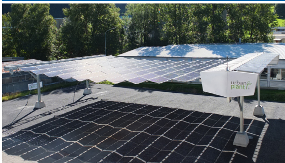
Fig. 1a Urban Plant horizontal –the PV modules are installed with an inclination of about 10° like in the 50kW prototype installed in Balzers FL [1]
