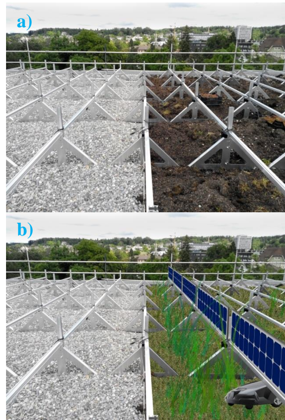
Figure 9: The PV power plant “Seniorenzentrum Wiesengrund” a) with vertical East-West facing bifacial modules before module mounting b) schematic of mounted bifacial PV modules and picture of the PV powered lawnmower working autonomously beneath the PV modules, located in Winterthur, Switzerland is a follow-up project of ZHAW with Solarspar and will be start operation on July 11 th , 2016.
