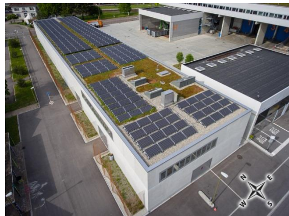
Figure 1: Aerial photo of the test facility with the installed PV capacity of 78 kWp located in Winterthur, Switzerland. All modules have an azimuth orientation of -3°.
