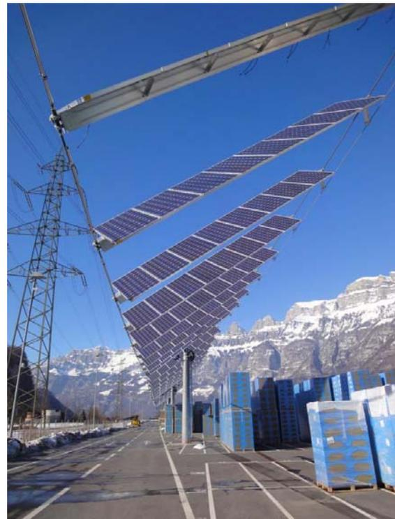
**Figure 7:** First Solar Wings 70kW two-axis tracking system installed at the Flumroc AG, Flums Switzerland and in operation since spring 2010.
