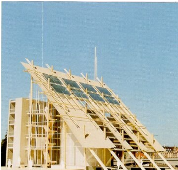
Figure 6: Municipal 50 kWp PV-filling station to be built by the City of Constance.
