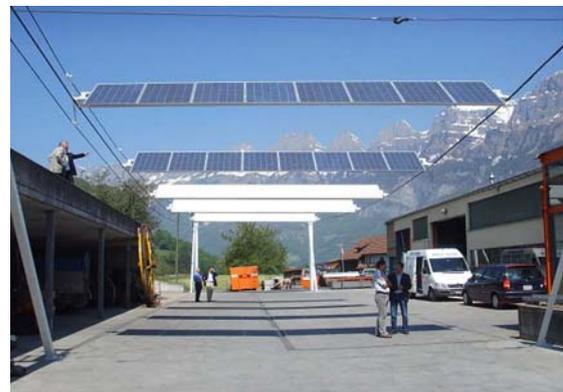
**Figure 3:** Solar Wings Prototype erected in Flums, Switzerland with a 40m distance between intermediate support pillars. This prototype version is equipped with horizontal PV module axis to allow the utilization of the space below the PV plant as a parking and loading area.
