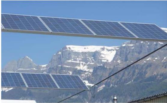
**Figure 4:** View of the steering cable turning details to rotate the PV plane around the beam carrier axis to follow the daily course of the sun.
